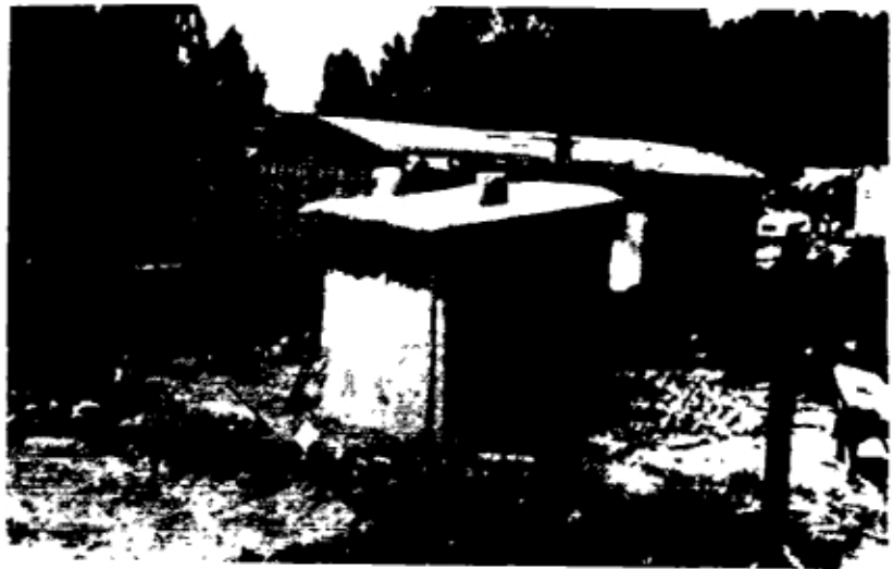
Photo 5: VIP with hessian-cement superstructure
