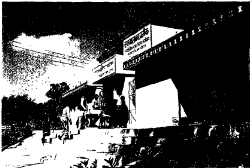
People entering in one of the Sulabh Complexes in Agra early in the morning for availing the facilities
