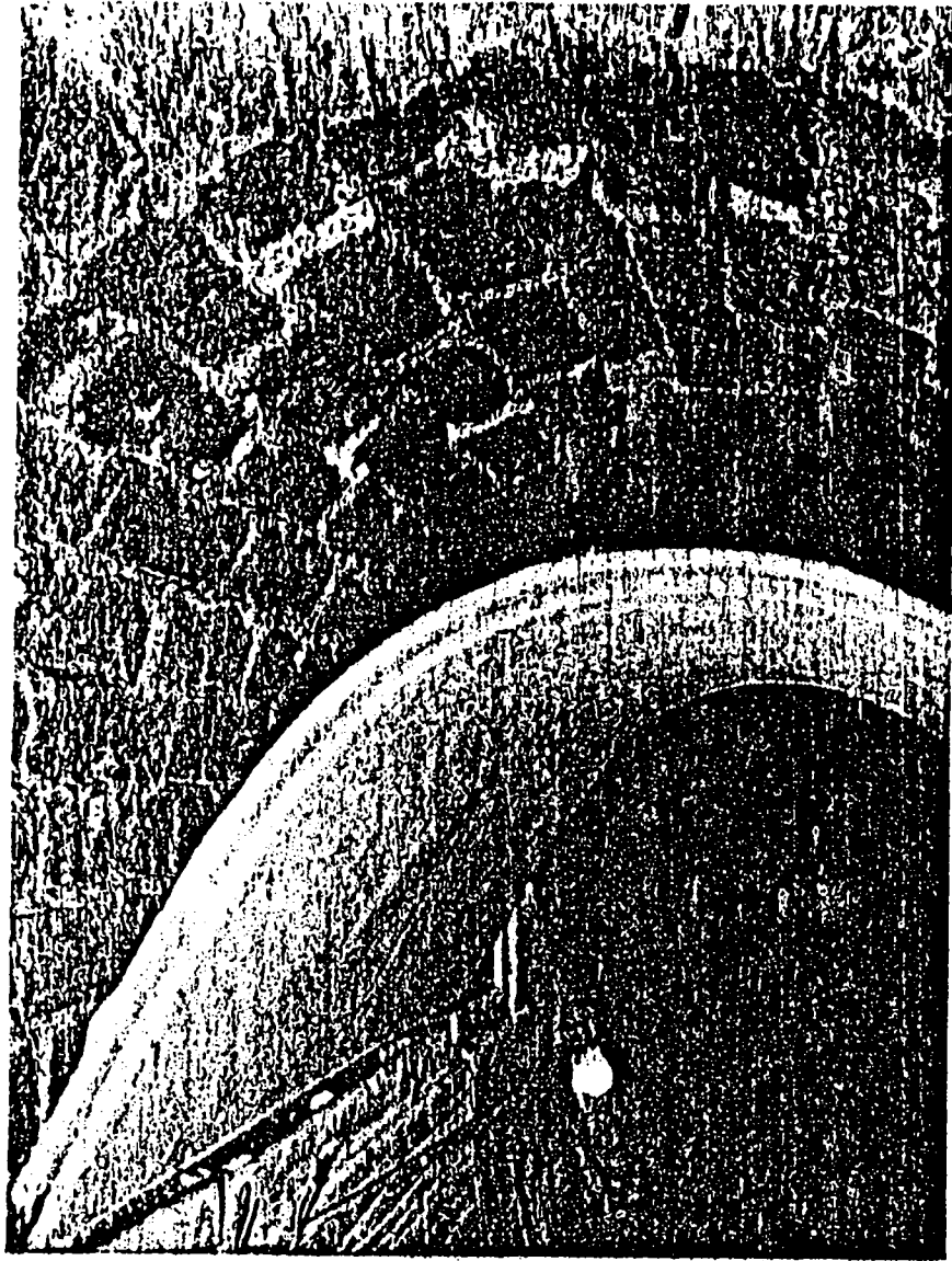
Fig. 12. Sewer lining with Charcon Composites GRC panels (Courtesy Transport and Road Research Laboratory)
