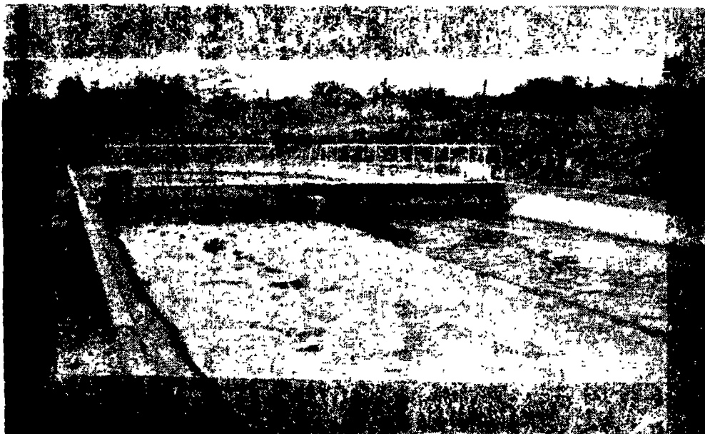
Fig 5. b) Oxidation pond.
