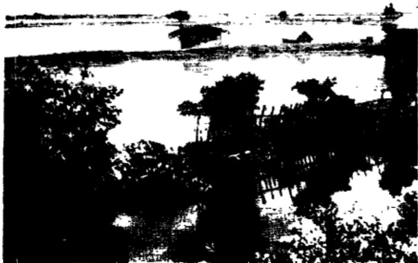
Figure 2.12 The Calcutta sewage fisheries (The canal in the foreground distributes raw sewage to the ponds.)
