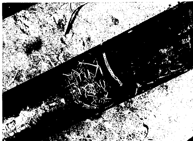
Fig. 8—The coating of this pipe, which was particularly mis-handled (the pipe was broken in half), has been deeply cut into, and the excess zinc (it seems) has been pushed back. This was the only pipe on which was found so deep a mark; however the basic metal has not been uncovered on any part of the barrel.
