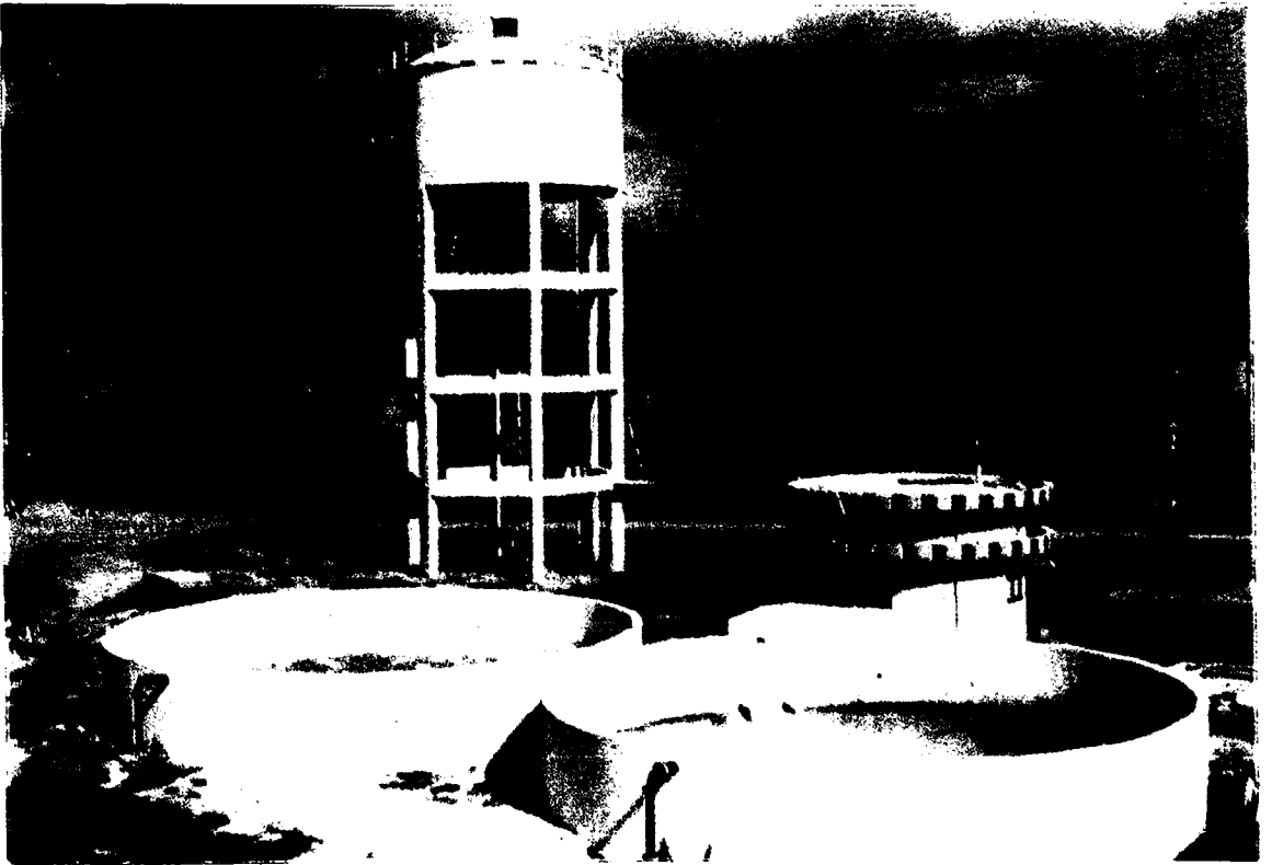
P.W.S. Scheme at Poluru Village of Yeddanapudi in Prakasham Dist. A.P.
