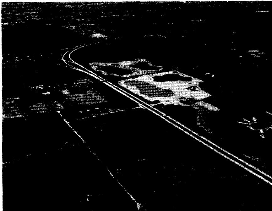
Aerial views of the completed Water Quality Management Project. The upper photo approaches from the north with the three marshes visible center right. The lower photo presents a southern approach, affording a panoramic view of the site and adjacent research areas utilized by other departments within the University.
