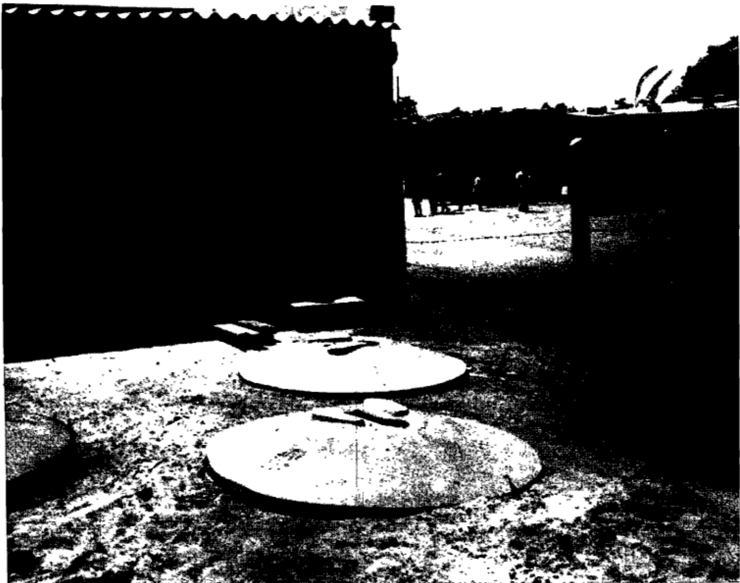
The new pit latrine slab requiring no reinforcement bars and a minimum of concrete, developed by Björn Brandberg, architect. Photo: Lena Hermansson
