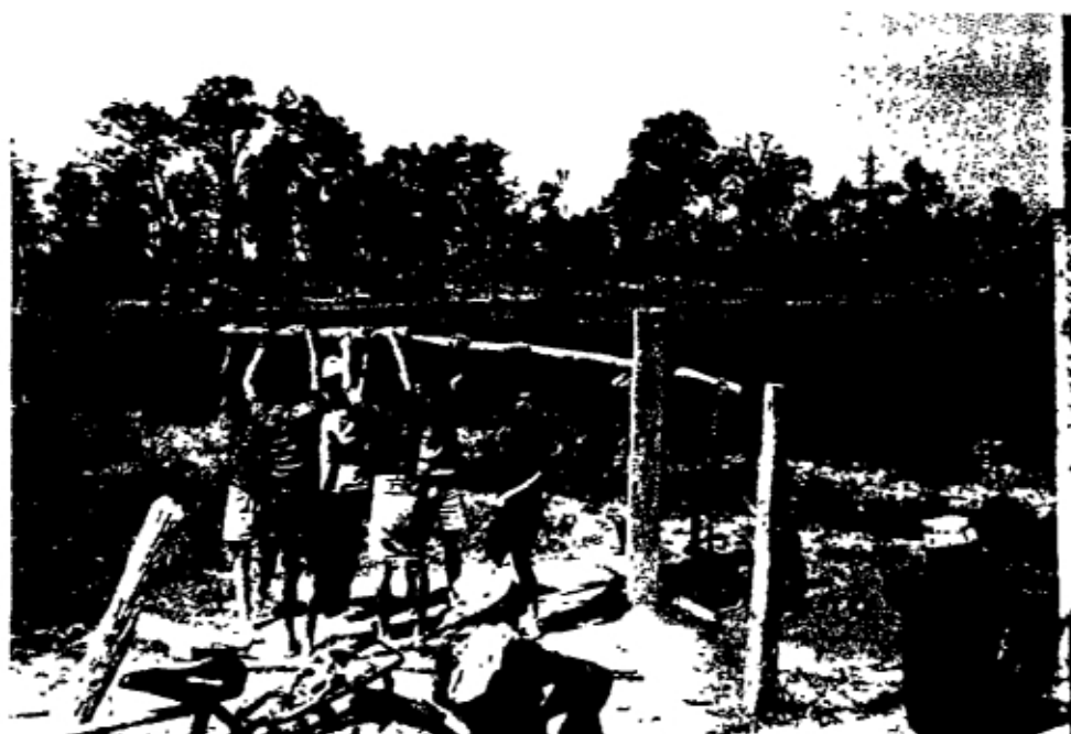
Photo 2. Men usually sludge the shallow tube wells.
