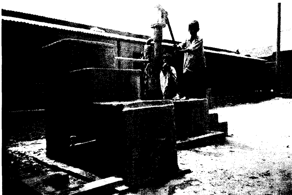
Figure 5.22: A tubewell sand filter (TSF) constructed in Sonargaon.
