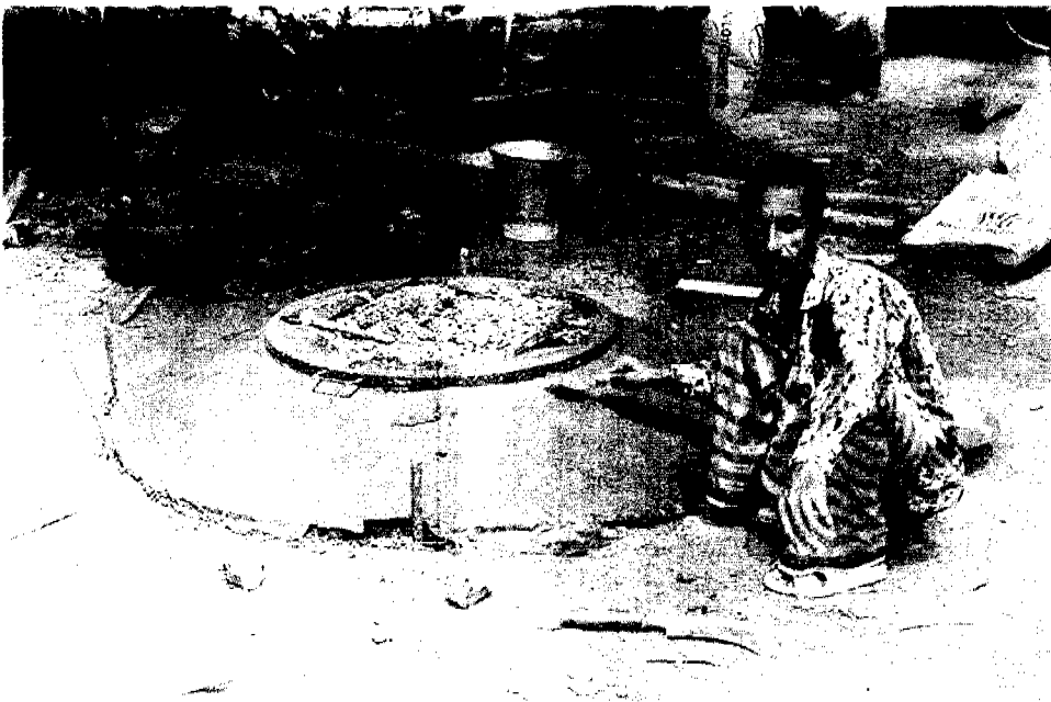
Fig. 5.8: Making of lids for the RWH.
