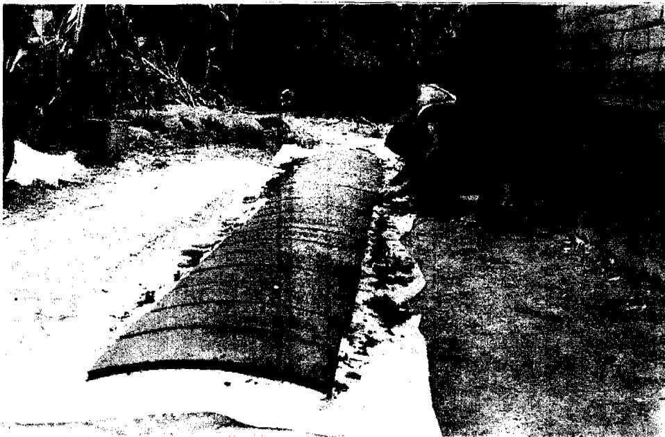
Figure 5.7: Construction of slabs for the 3200 litres RWH.
