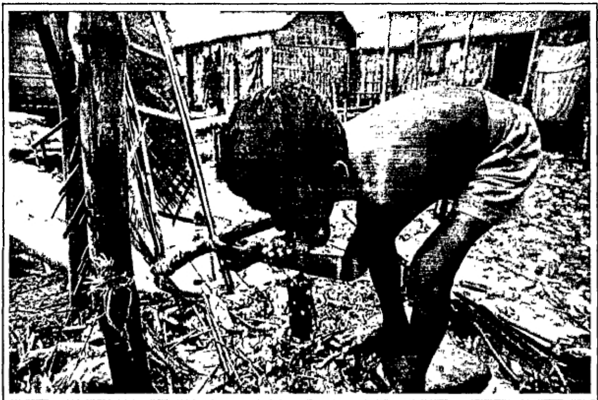
8. A water point in Bijili Mohalla slum. Probably an illegal connection, it has no tap, washing platform or drainage (photo for WaterAid by Jim Holmes).
