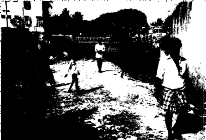
Foot path work in progress
