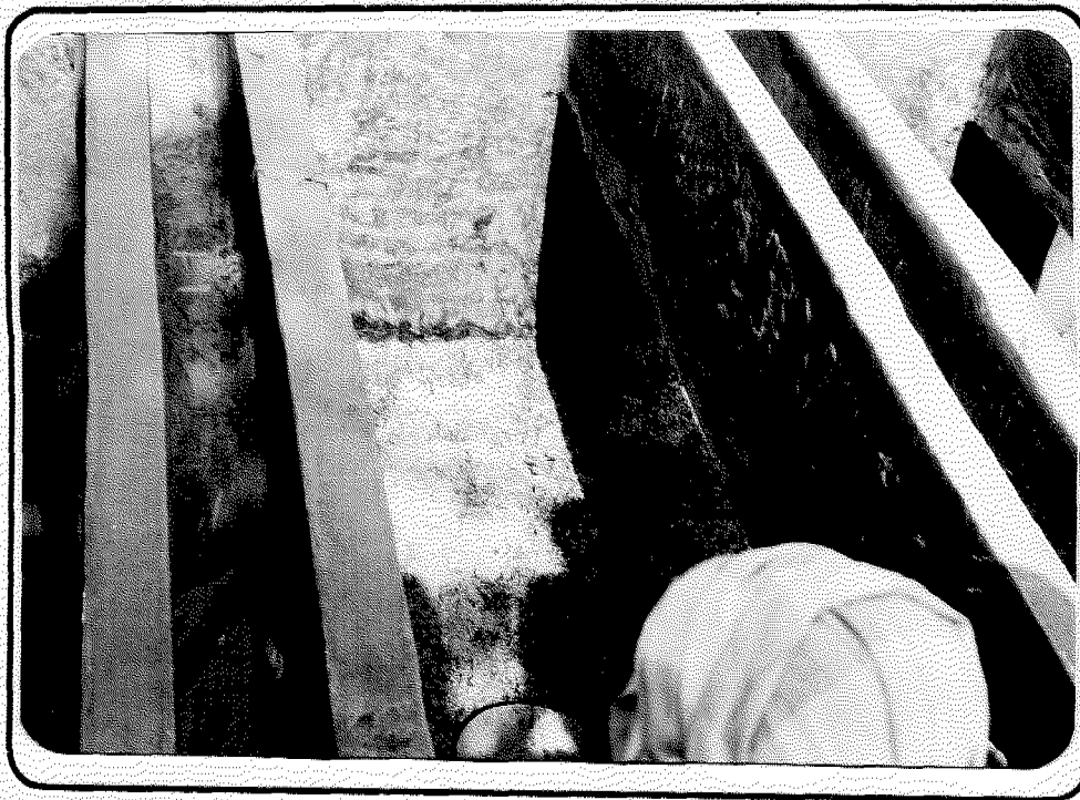
A SAND FILTER WITHOUT FILTER SAND !
