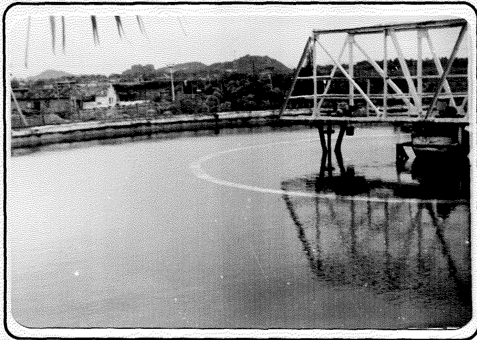
CLARIFIER FLOODED DUE TO OVERLOADING - NOT AN UNCOMMON SCENE
