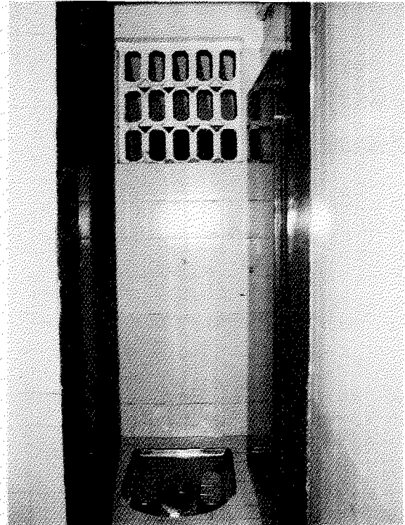
Stainless pans, used in some Sulabh toilets, are easier to keep clean than the ceramic ones
