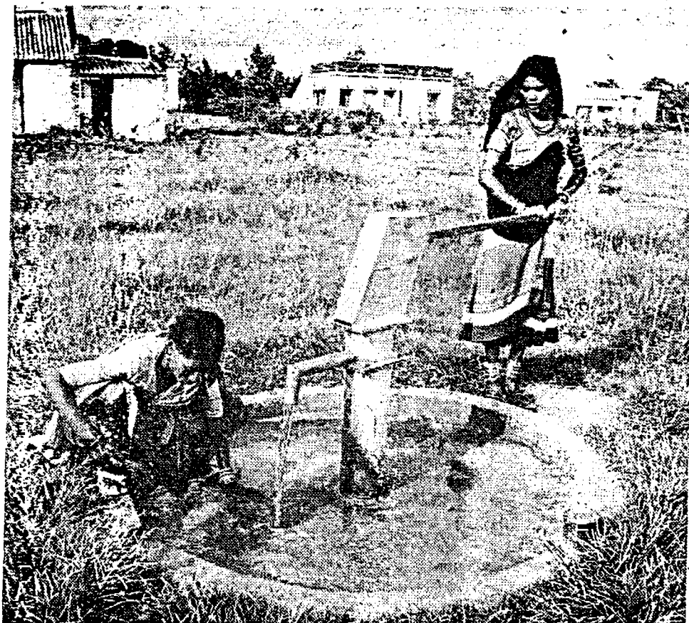
Keeping the pump base and surroundings clean.
