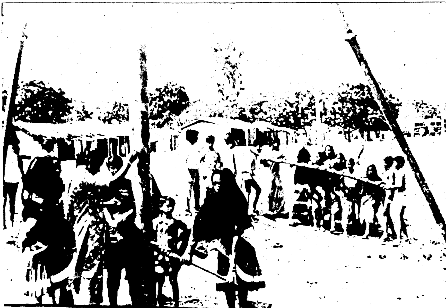
WOMEN LEARNING BORING PROCESS AND HANDLING OF PIPE ASSEMBLY OF INDIA MARK-II H.P.
