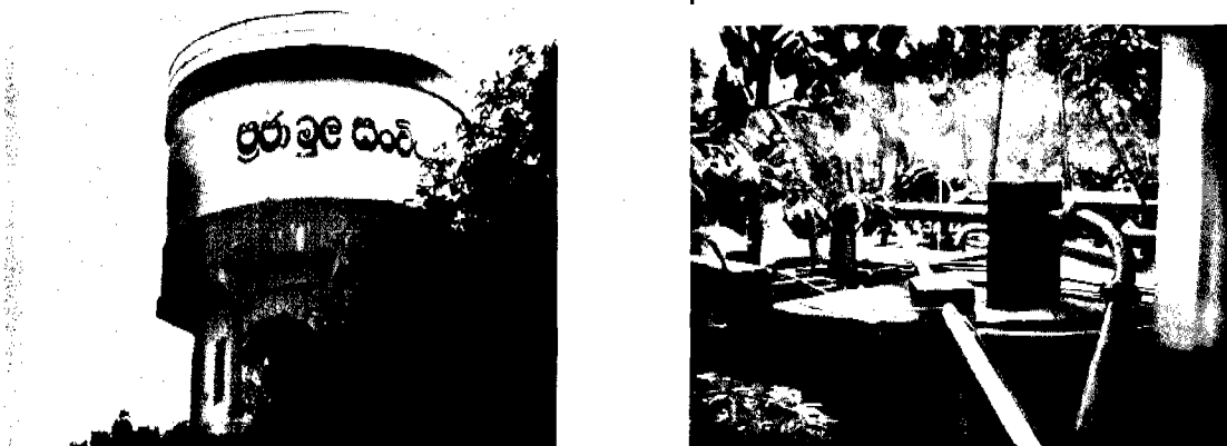
Figure 4.36: Water tower and intake well of Kuruwita water supply system.
