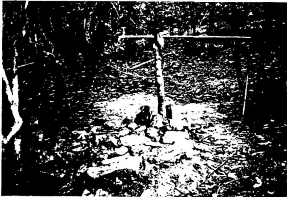
BELO/NJINIKIJEM: Standpipe of extension (done by population). One of the largest CD/HELVETAS WS systems; constructed 1971-80; gen.rating 3; ref.no.52.
