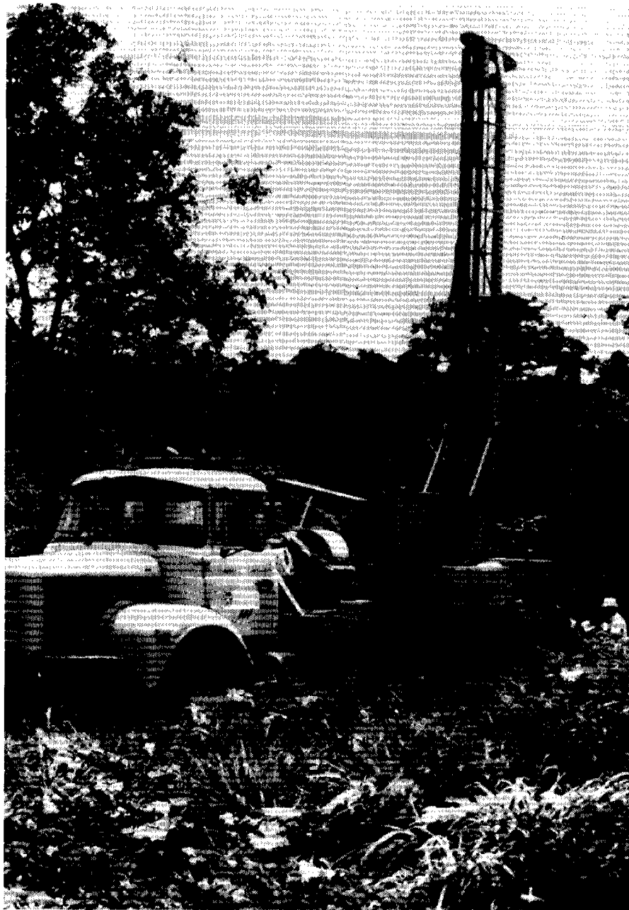
Figure 7: Well drilling involves considerable cost.
