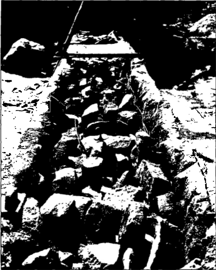
Photo 10. Constructing wall with rock filling
