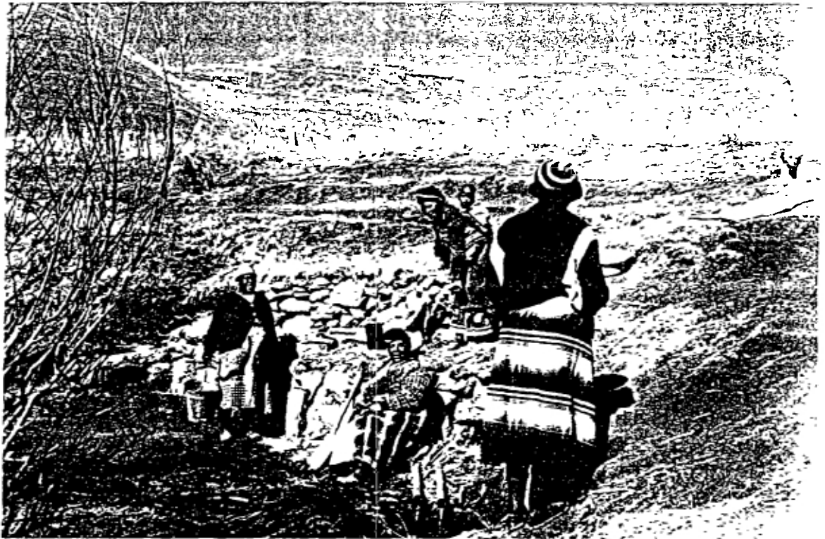
4. A nearly completed protected spring
