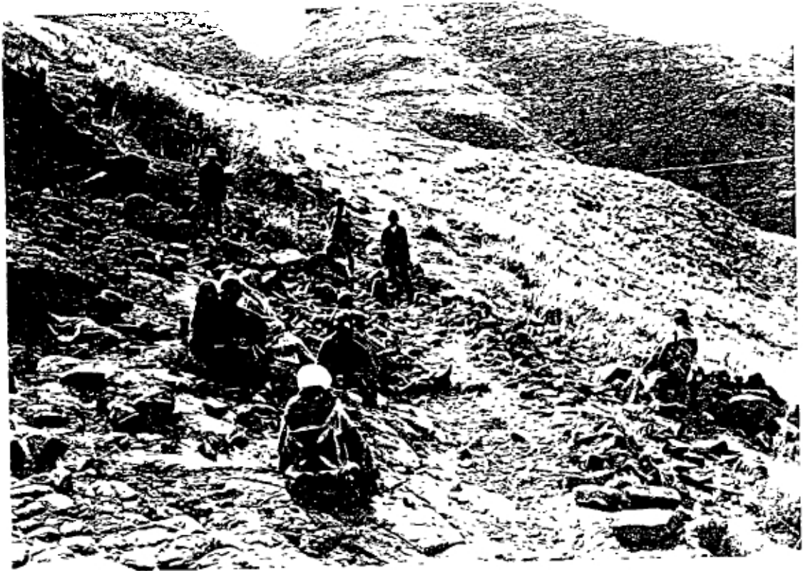
5. Villagers breaking stone for concrete
