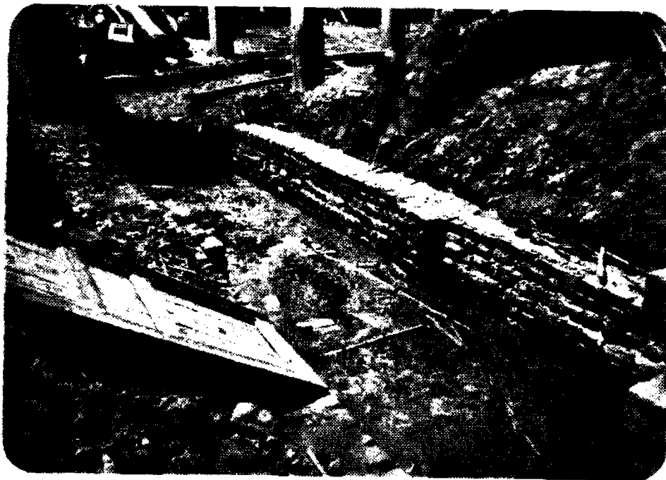
Illustration 6 Standing water in foundation excavation
