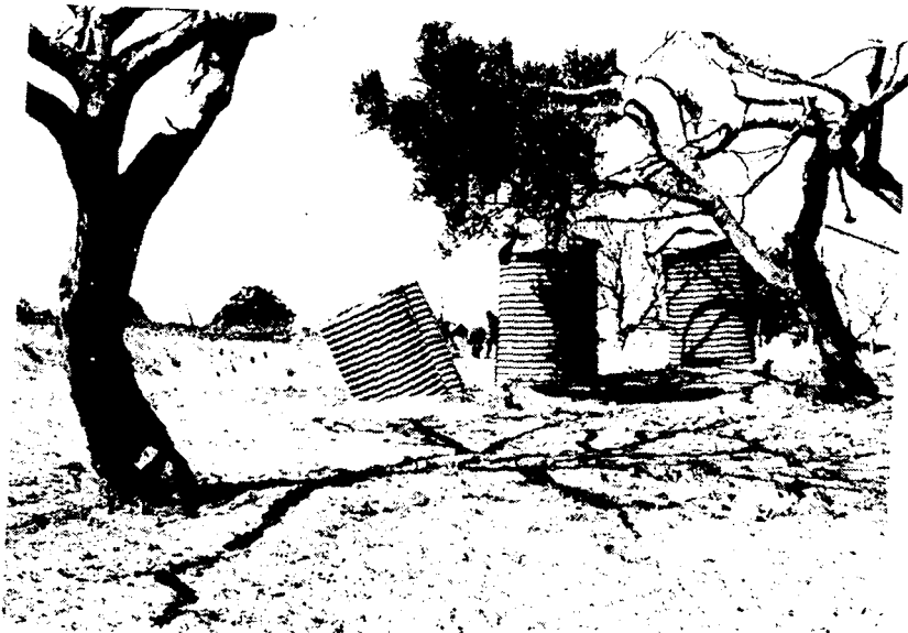
Figure 6: What happens if there is no diversion furrow round a toilet to divert surface water and if the slab is too small for the pit. Surface water can erode away the collar of the pit.
