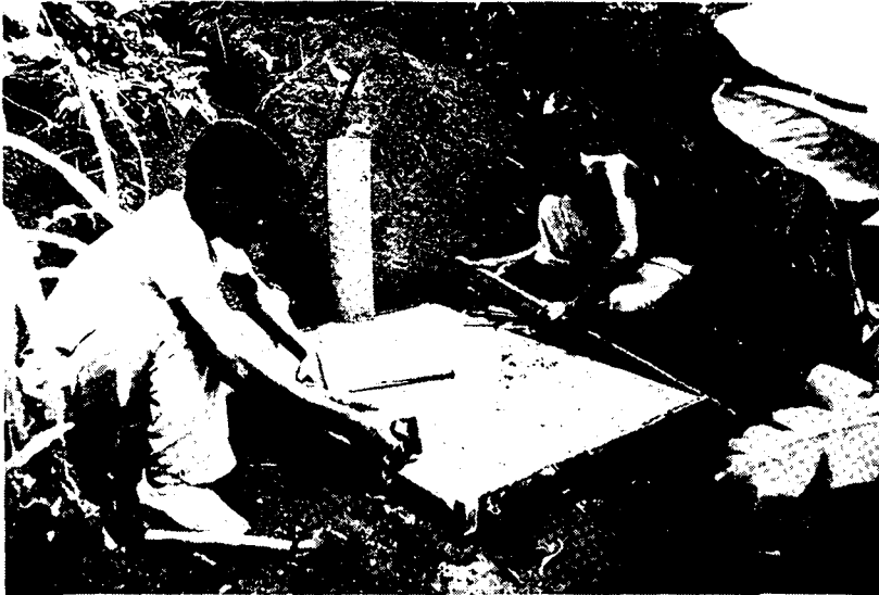
Figure 1: A good example of a spring protection tap and splash plate being constructed by trainees. The V-Box is approximately 12 metres away.
