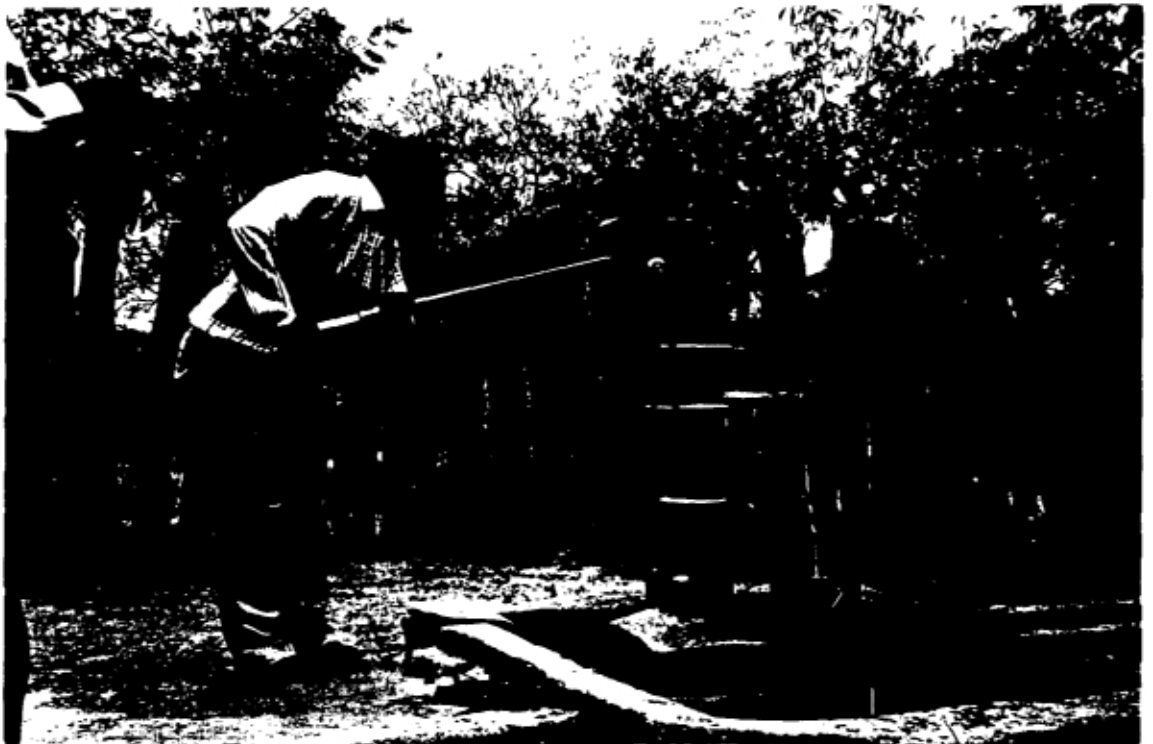
PLATE 5: PROTECTED WATER SOURCE AT SIMALELE VILLAGE
