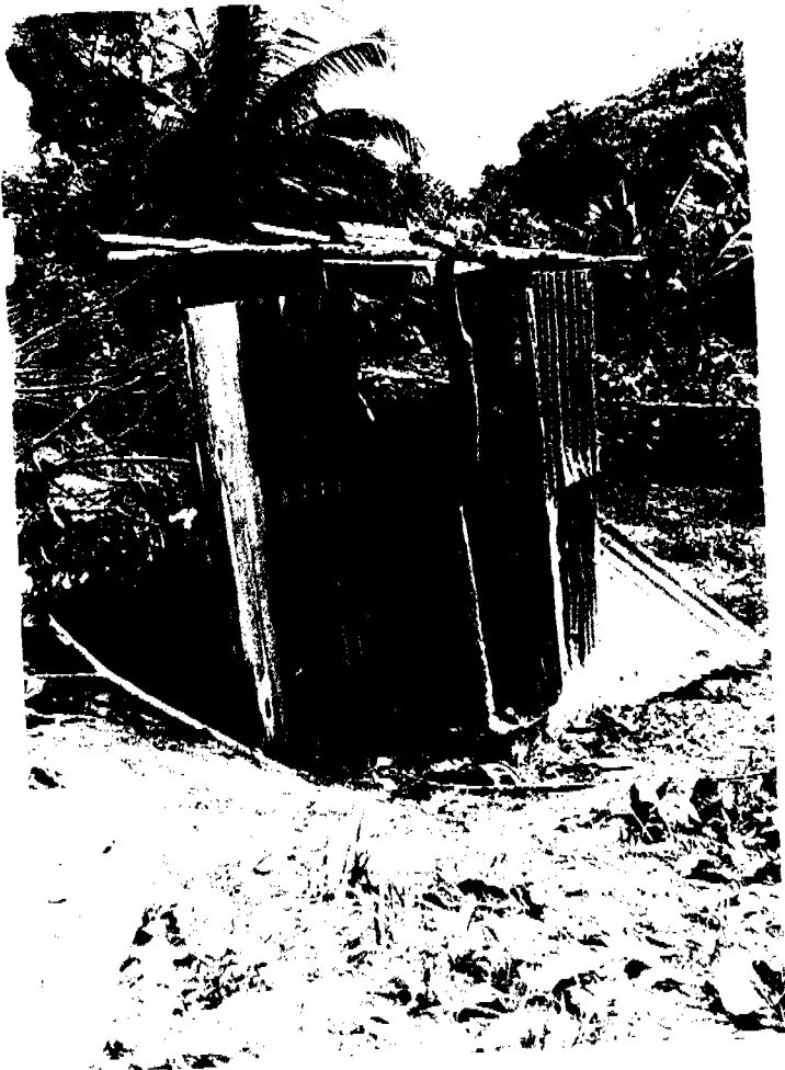
Pit Latrine that needs to be repaired in Woodside.
