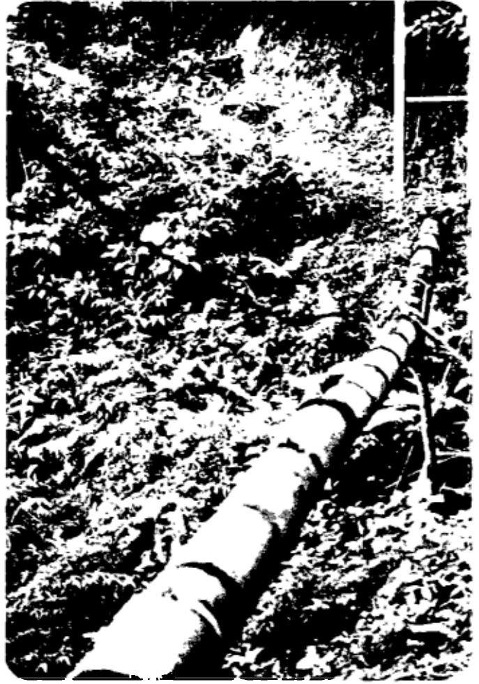
PHOTO 8. PVC Pipe Bridge. Note deflection at the center of the span.
