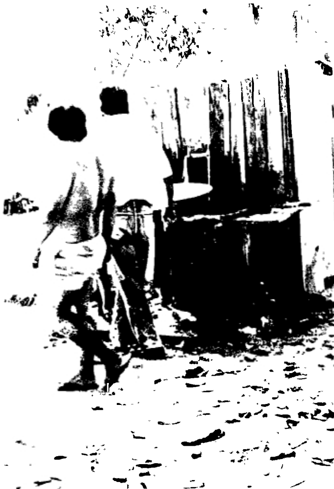
PHOTO 4. House Tap and Shower. Note poor drainage on the floor.
