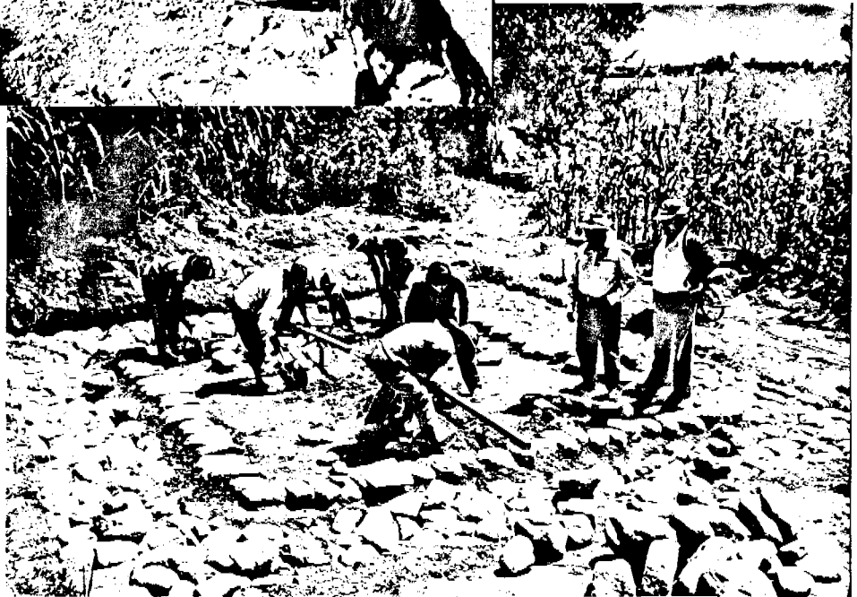
Masonry storage tank under construction.
