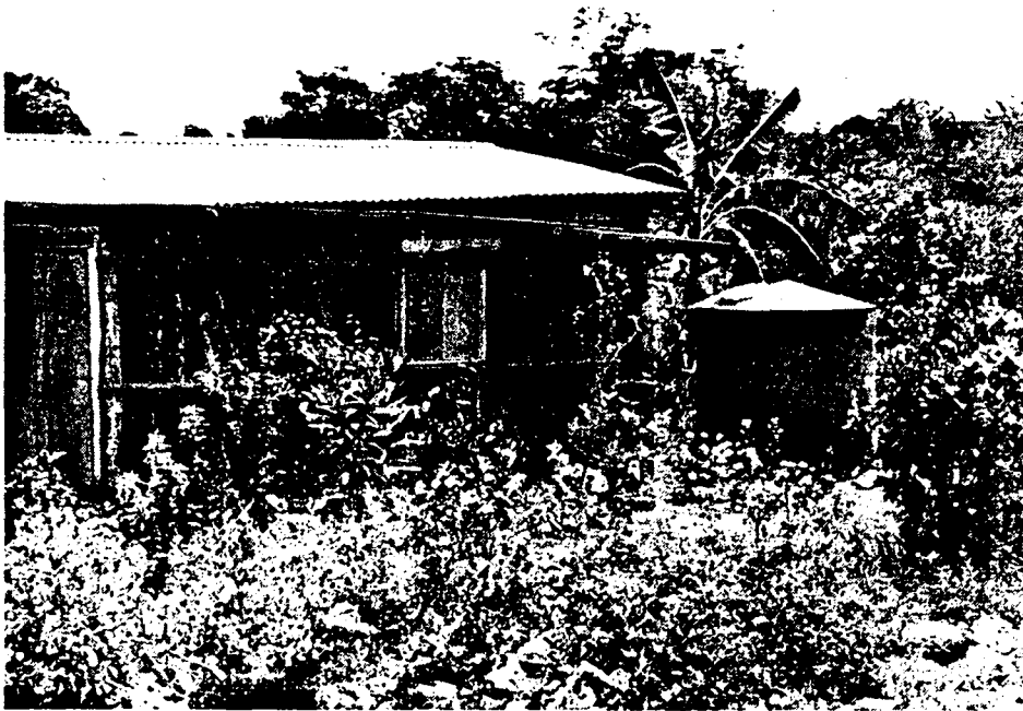
Figure 11. Typical rural rainwater catchment system.
