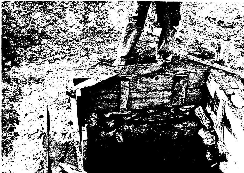
Figure 4. Construction of latrine collar.
