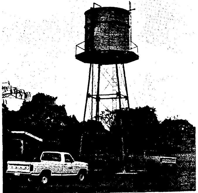
Figure 12. Elevated water storage tank from previous CARE project in Douglas.
