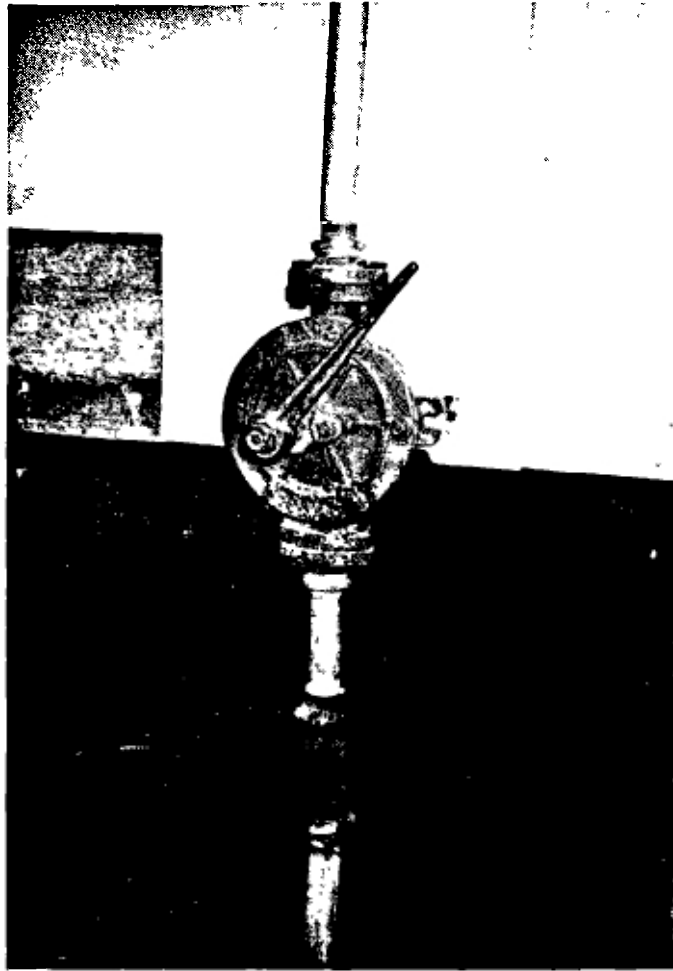
Photo 22. Semi-rotary handpump.
