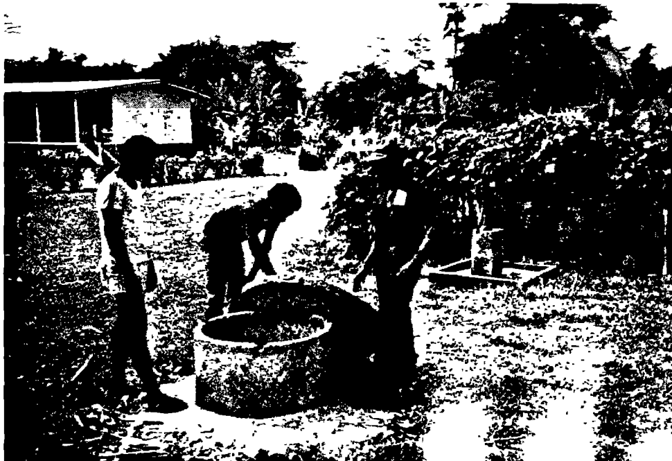
Photo 8. Dug well and offset handpump.
