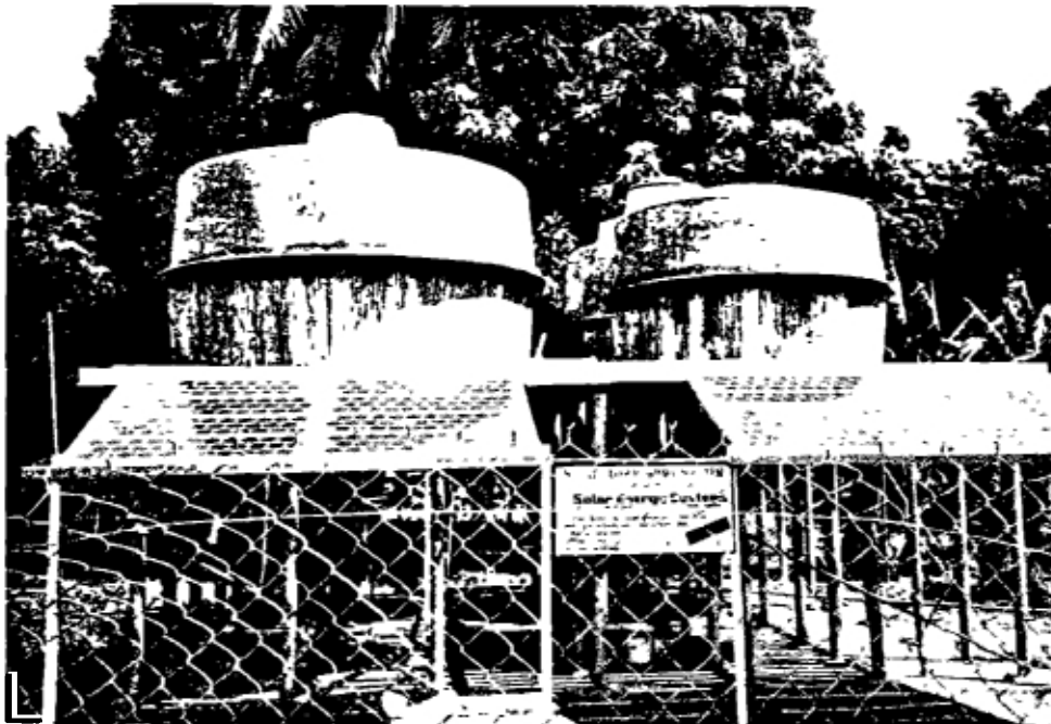
Photo 5. Fiberglass tanks and photo-voltaic panels.
