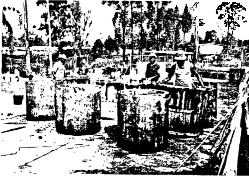
Photo 7. Production of well liners.
