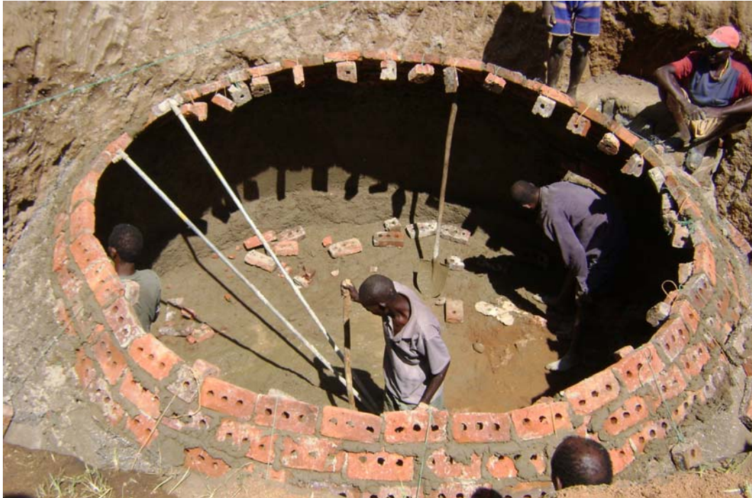
Digester for bio-gas latrine under construction, Konso
