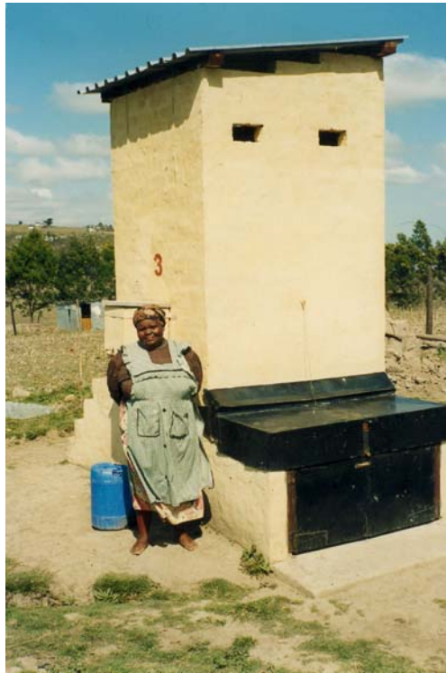
Figure 3: Completed urine diversion toilet unit at Sinyondweni
