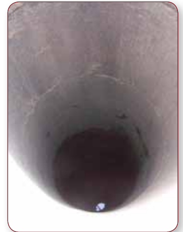
This is an open hand-dug well in Tantiaka targeted to be sealed, purified and given a rope pump for greater ease of use.
