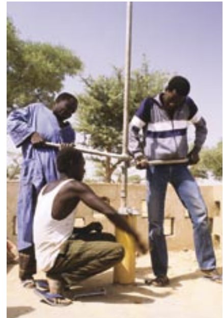
Low-cost hand-drilling technique
