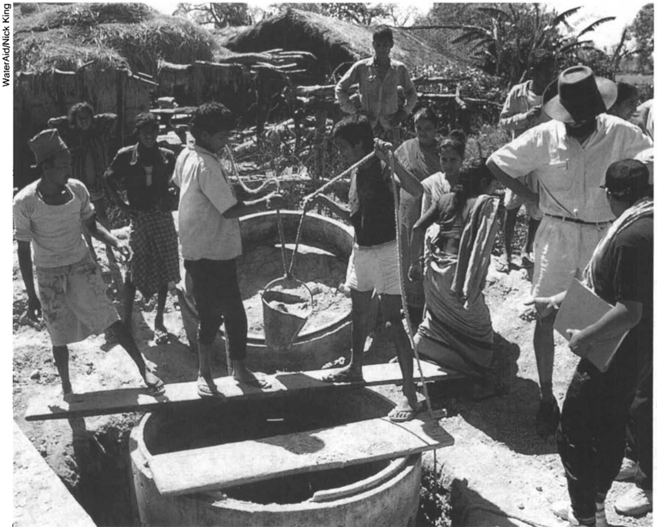
A concrete-lined well needs external resources and technology, but is much cheaper than a borehole.
