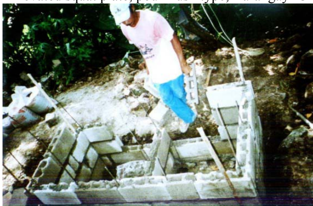
Construction of vaults for EcoSan toilet using hollow blocks
