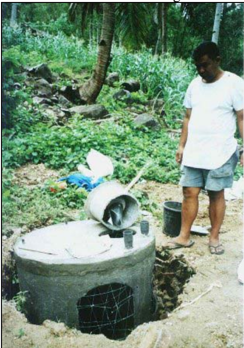
Construction of processing vaults and movable toilet bowl
