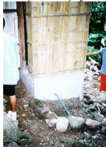
Drain of urine collector ending above plant bed
