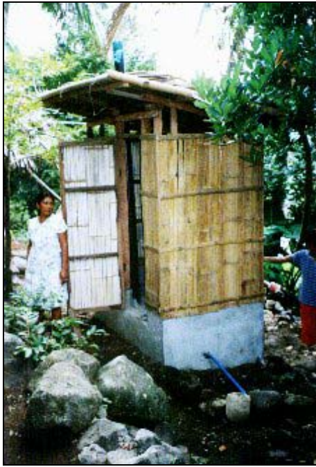
Completed EcoSan toilet in Barangay 14
