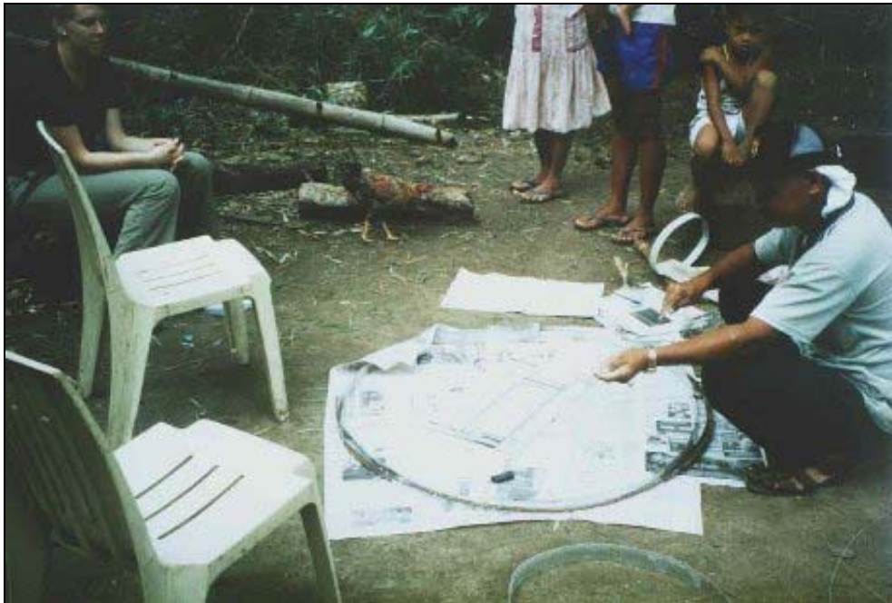
Making the slab using ferro-cement technique
