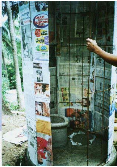
Construction of superstructure
