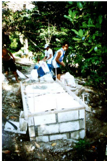
Preparations for construction of toilet floor using cement
