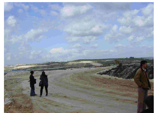
Pathway cleared to make way for the wall. Photo courtesy PENGON.
