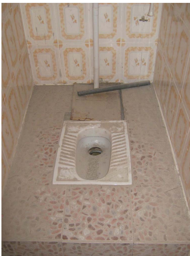
New build toilet facility that was to be opened within days of the team visit.
