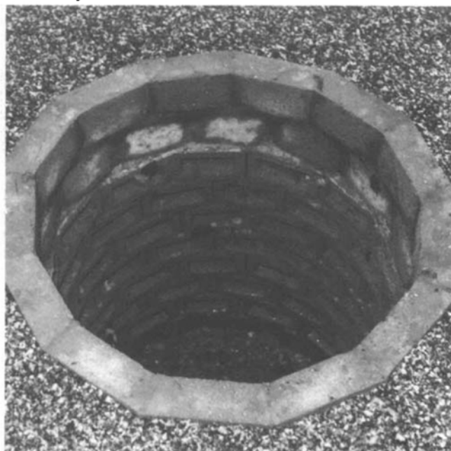
A lined percolating pit, using purpose-made concrete blocks.
