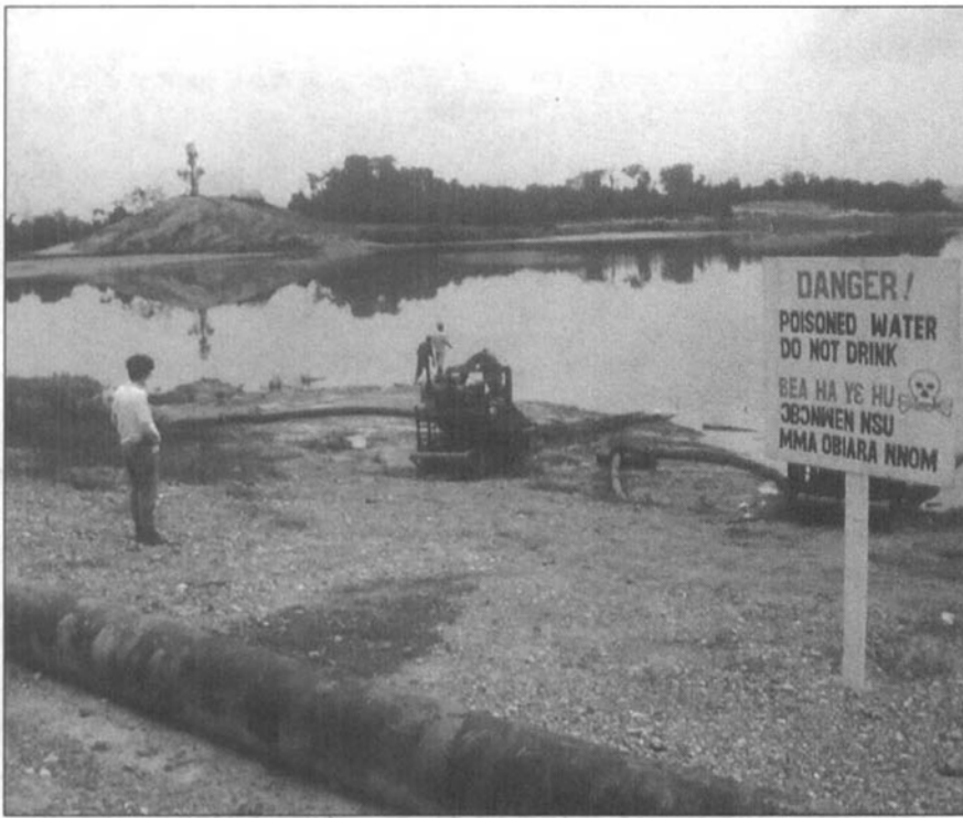
Hazards associated with mine water tailings lagoons must be clearly identified to prevent use by local people.
