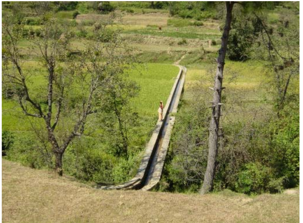
Improved traditional irrigation scheme, India
