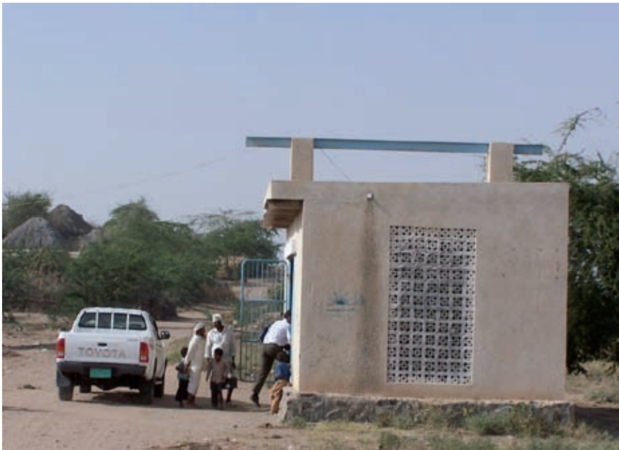
Pump house, Dir Al Maqboli, Hodeidah Governorate
