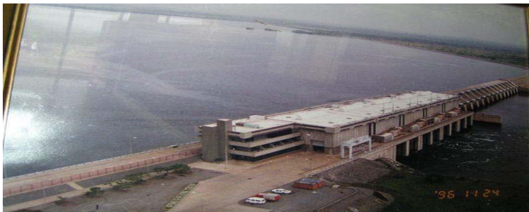
Figure 1.14: An Aerial View of the Kpong Dam Site
