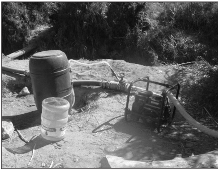
Suction side-dosing arrangement
