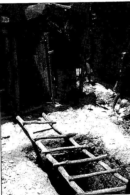
As one latrine pit fills up, a new one is dug.
