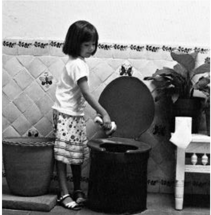
Figure 6: Urine-diverting toilet in a Mexican home
