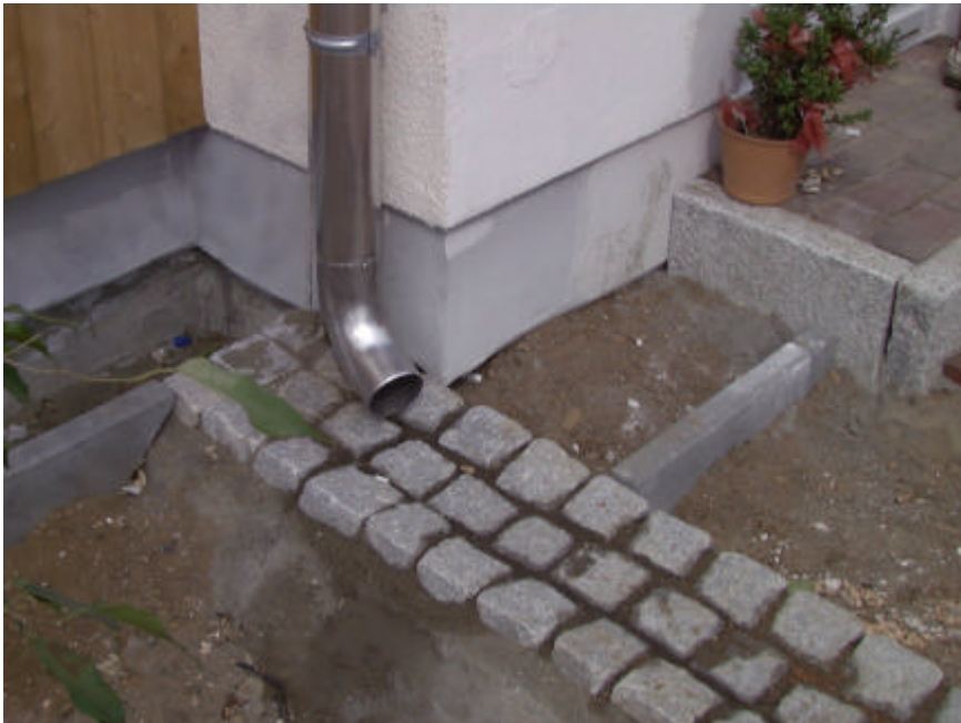
Fig. 5: Gutter for the transportation of stormwater
