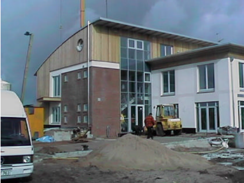
Fig. 4: Community building of the residential area Lübeck-Flintenbreite
