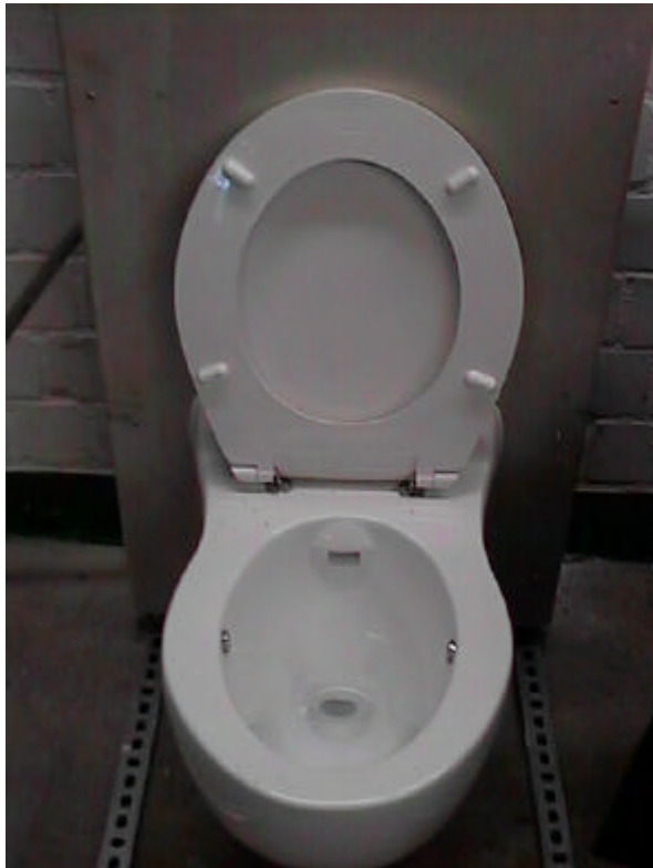
Fig. 3: Vacuum-toilet flushing with approx. 1 l per flush
