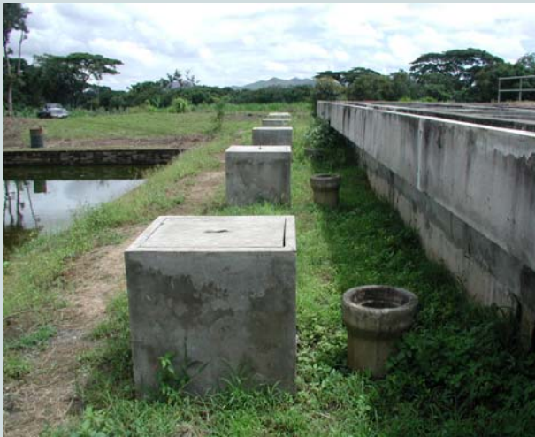
Sludge evacuation system at the Imhoff tank, Masatepe, Nicaragua. Source: Martin Gauss, 2005.
