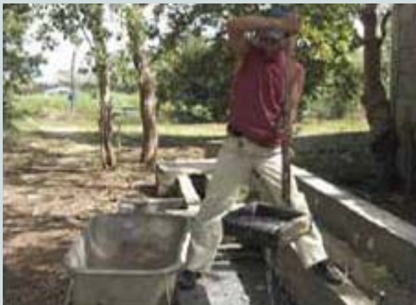
Cleaning the inlet channel. Source: WSP, 2006.
