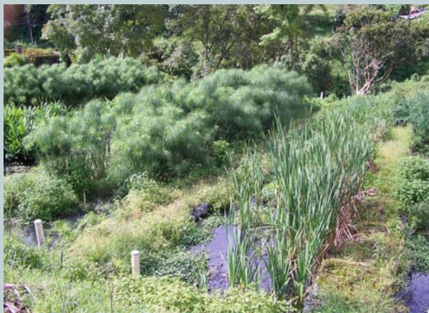
SSHF constructed wetlands for tertiary treatment in Pereira, Colombia. Source: WSP (2007).
