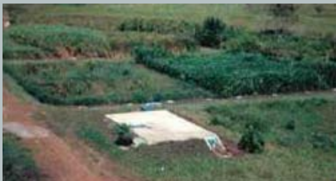
SSHF constructed wetland system at Masaya, Nicaragua. Source: Proyecto Biomasa, 1997.
