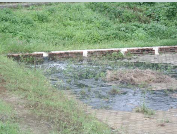
Sludge drying bed at Masatepe, Nicaragua. Source: Martin Gauss, 2005.
