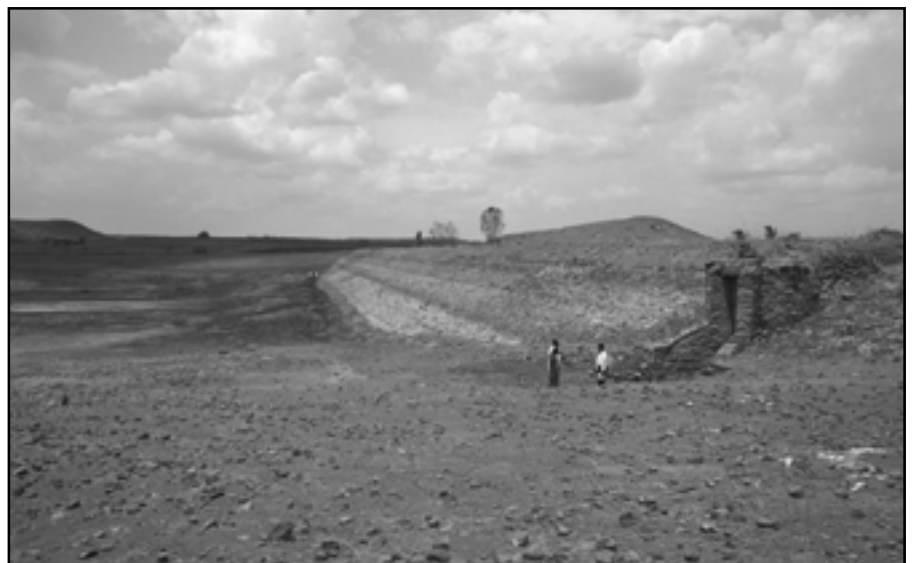
This tank is dry partly as a result of water harvesting upstream
