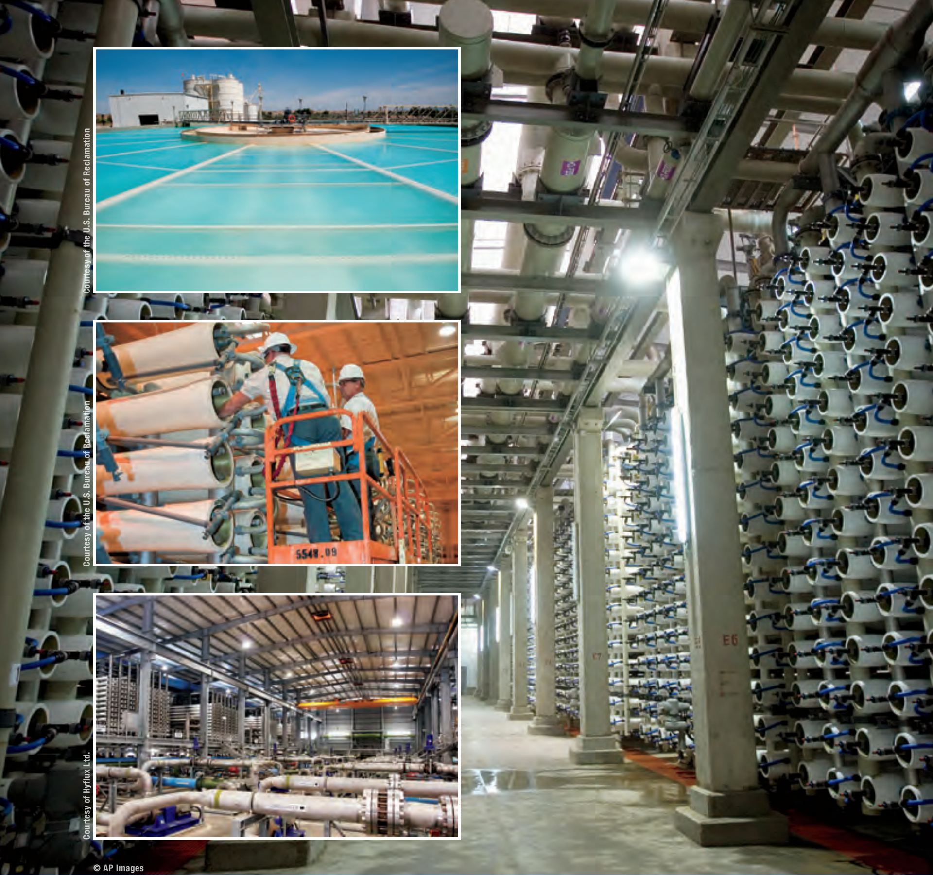
Above: The desalination plant in Hadera, Israel, is the third of five planned facilities expected to provide one-third of Israel's drinking water. (inset top and middle) In Yuma, Arizona, one of the world's largest reverse osmosis plants is used to reduce the salinity of the Colorado River. (inset bottom) The SingSpring desalination plant in Singapore is a seawater reverse osmosis plant that produces up to 136 million liters of drinking water per day.
