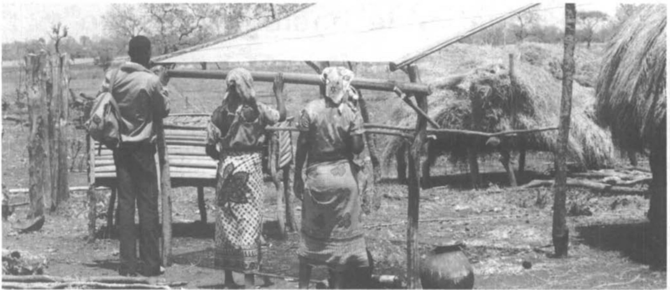
Storage vessels are placed below the lower corners to catch the run-off.
